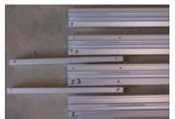
Install pre-drilled splice box aluminum as shown in below picture. Use (4) ¼" x 1 ¾" Truss head bolts and (4) ¼" lock nuts. On splice bars match corresponding letters to face each other. (A to A, B to B, etc)
